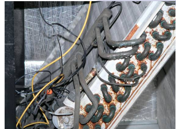
Corroded Air Conditioning system due to Chinese Dry Wall – image courtesy of chinesedrywall.com
